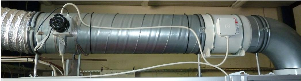
Figure 4.14.: Photo of the ventilation part including the fan (right side) and ventilation monitoring (left side). The system is connected on its very left side to the exhaust to the ambient outside the lab.
